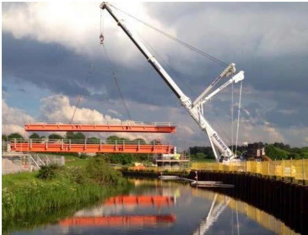
Photo 2: Temporary Bridge – Typical Installation
