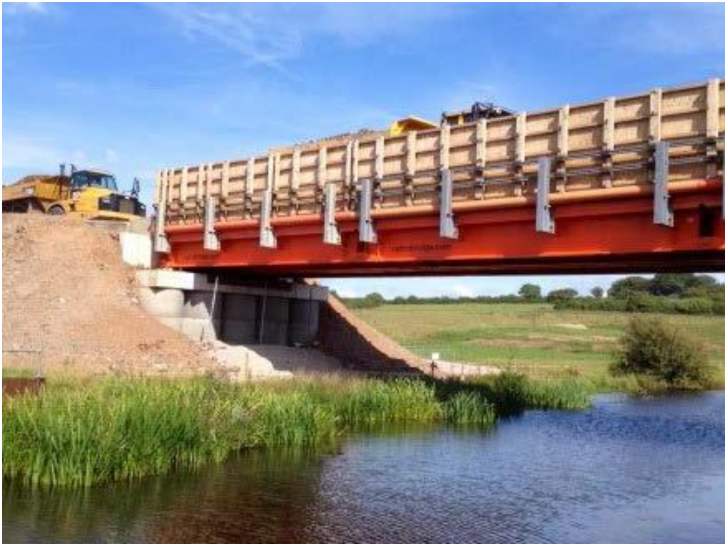
Photo 1: Temporary Bridge – Typical View
